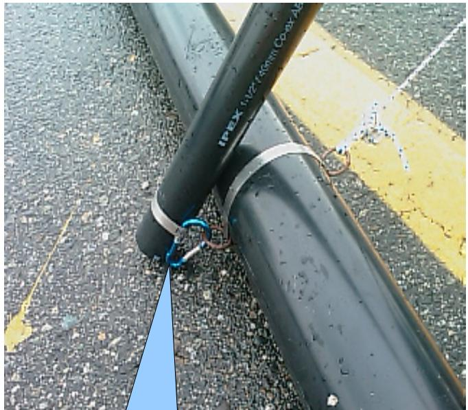
Carabiner clamped to upright connects to ring on outside of 4 inch pipe
