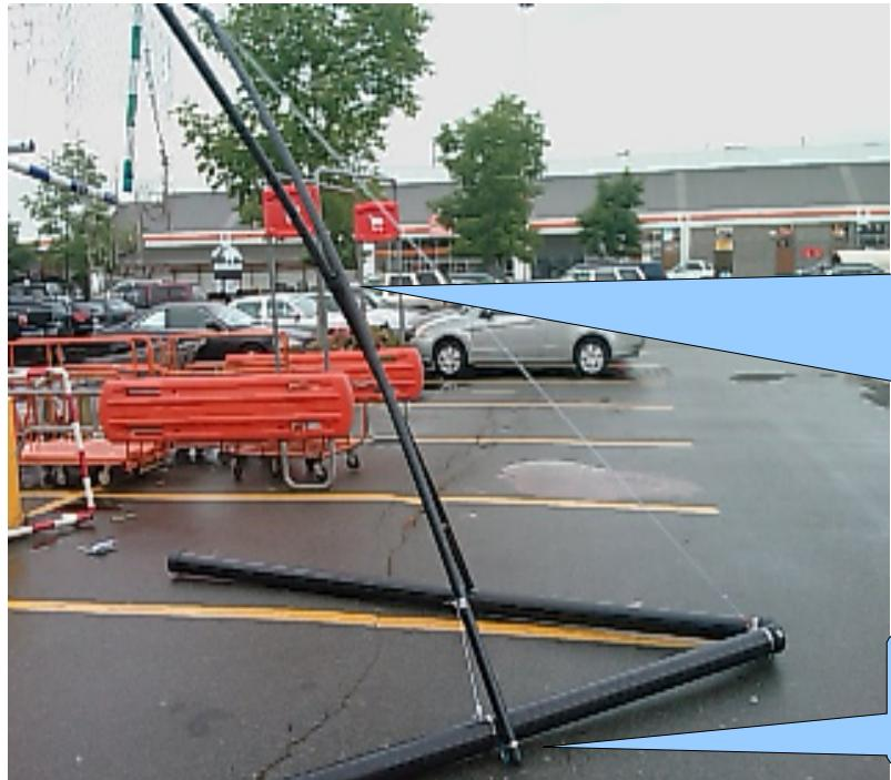
pin uprights together with bolt – find this place by setting it up first, then tape, then drill hole, bolt not tight, allow to scissor
